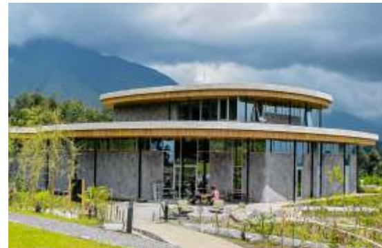
This end-to-end participatory process results in high quality, affordable and healthy buildings.
