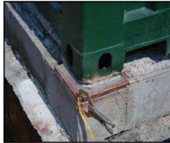
Figure: Illustration of Welding Container Column To Plate
