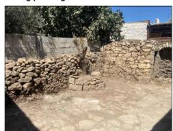
Demolishing Stone Wall, Brick, Planter, Sultani Tiles, and Outdoor room with numbering the stone of the room to rebuild it again
