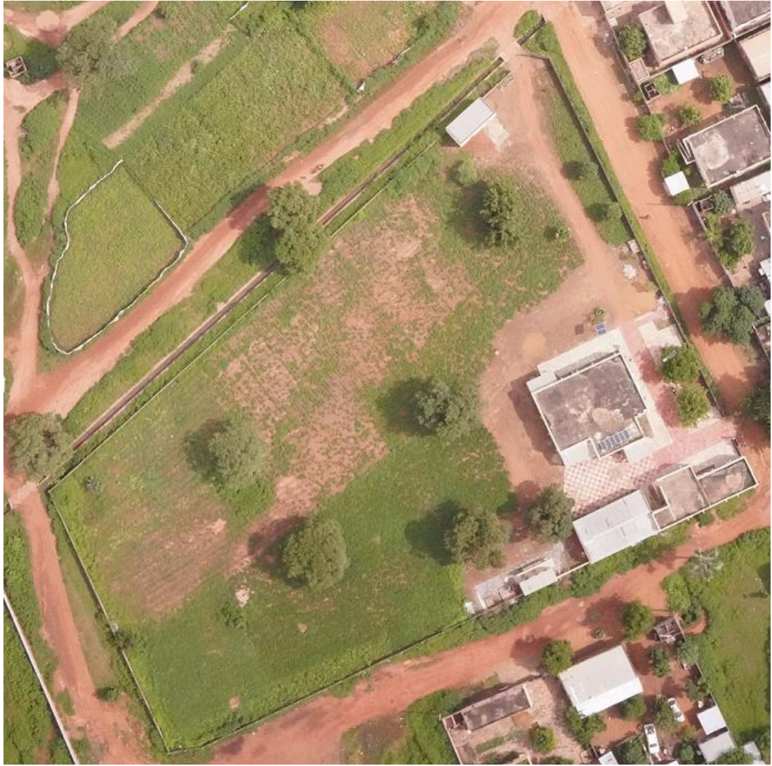
CSCOM de Souban (12°50'58.0"N 7°34'54.1"W)
