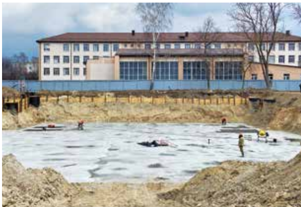
Construction of a shelter in Baryshivka, Kyiv region. © Enabel
