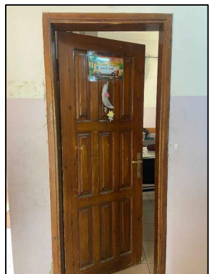
Fixing wall and painting of wooden doors
