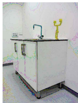
New 10 cm Block wall
