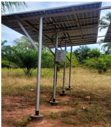
Solar panel mounting structure / and Ant climbing
