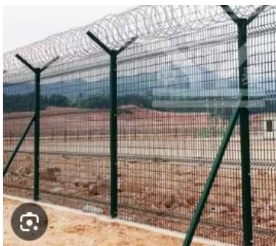
Sample of 75mm thick treated fence steel post fixed with razor wire and barbed wire on top
