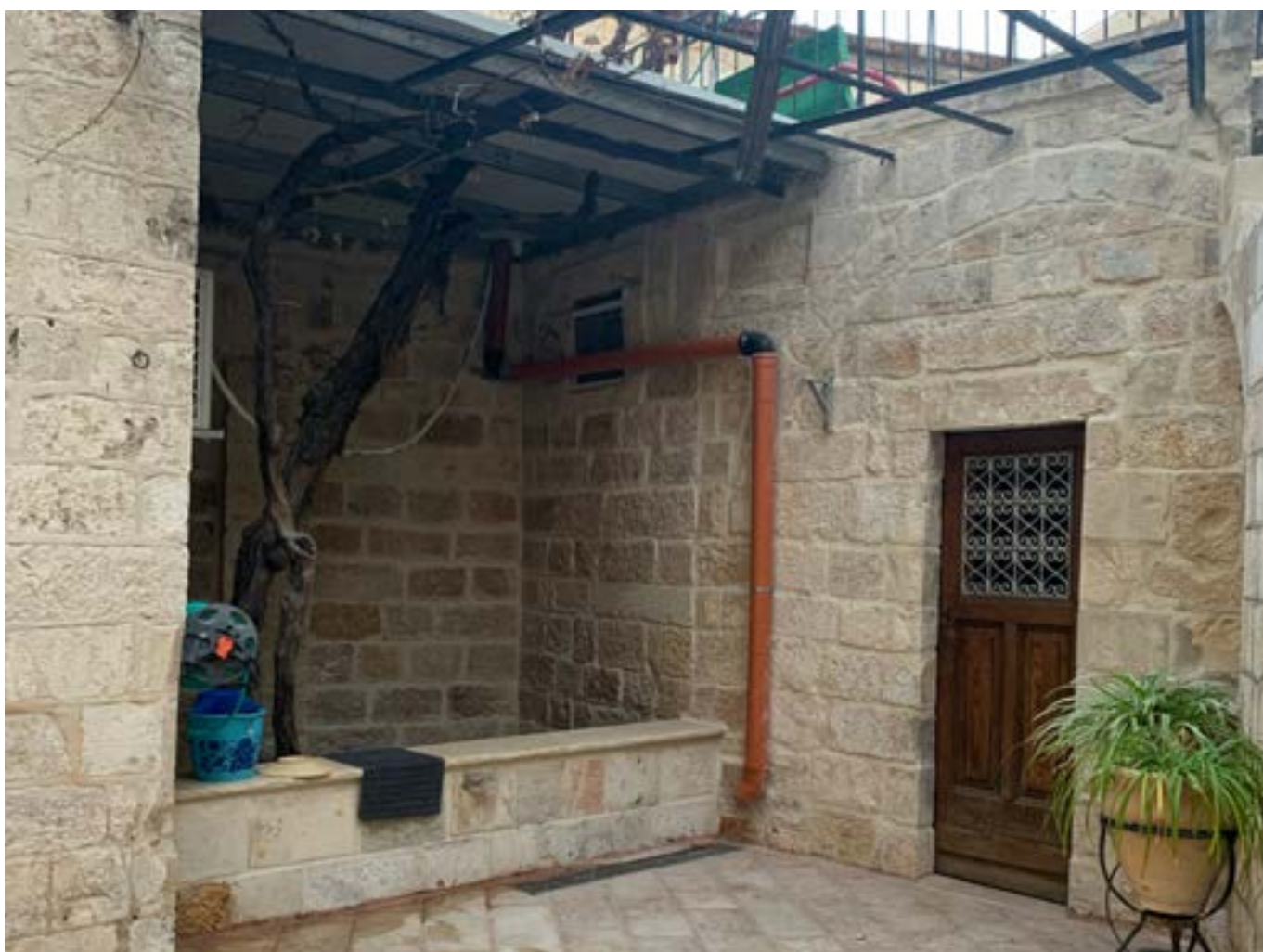
Actual state of courtyard Room 6, view from the terrace upstairs - P&R
