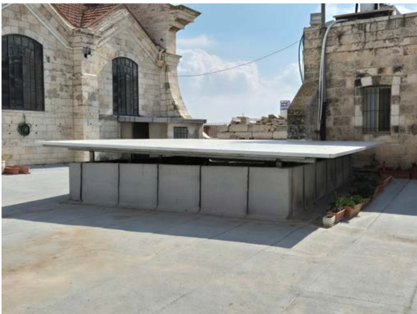
Actual state of courtyard Room 4, view from the roof - P&R
