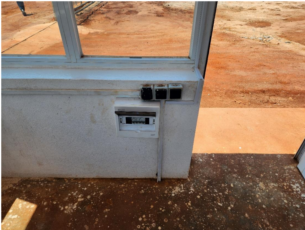
Figure 10: Electrical board in the guard house
