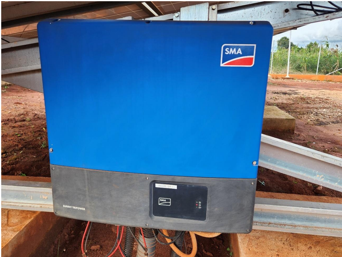
Figure 4: Photo of the solar PV inverter to replace in Mugulama mini-grid
