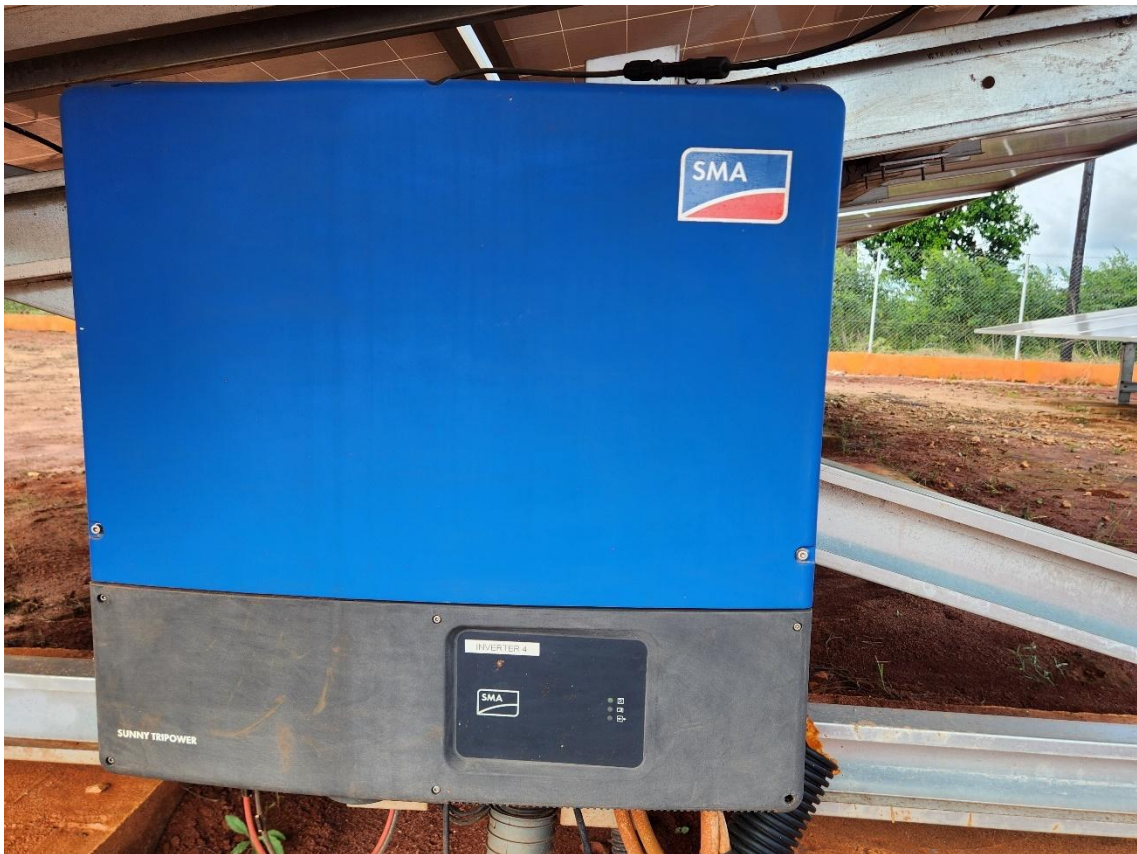
Figure 5: The solar PV inverter for which the communication board should be replaced
