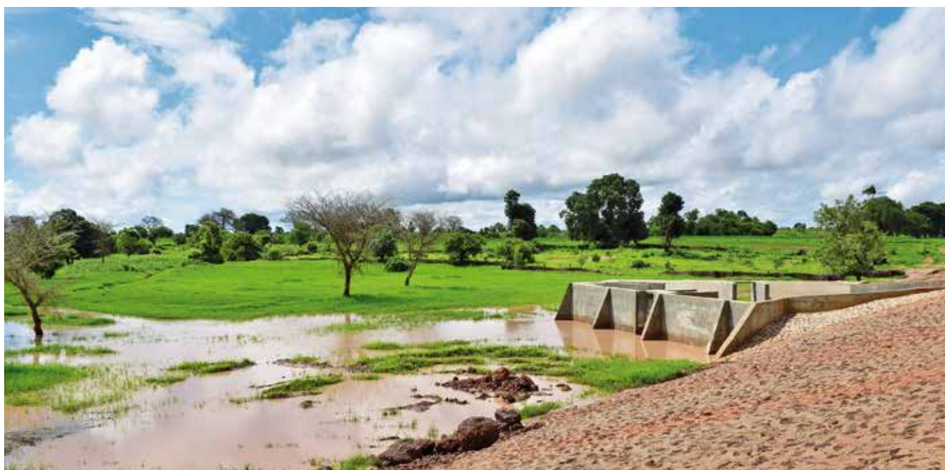
Kayemor (Kaolack), retention and overtopping dam. Photo: © BTC / Marcella Pasotti
