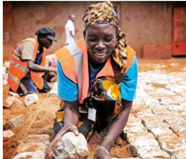
Bujumbura: Paving is easy to maintain and more sustainable than asphalt or concrete roads. © BTC / Rosalie Colfs
